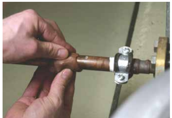
Sealing of a copper tube
